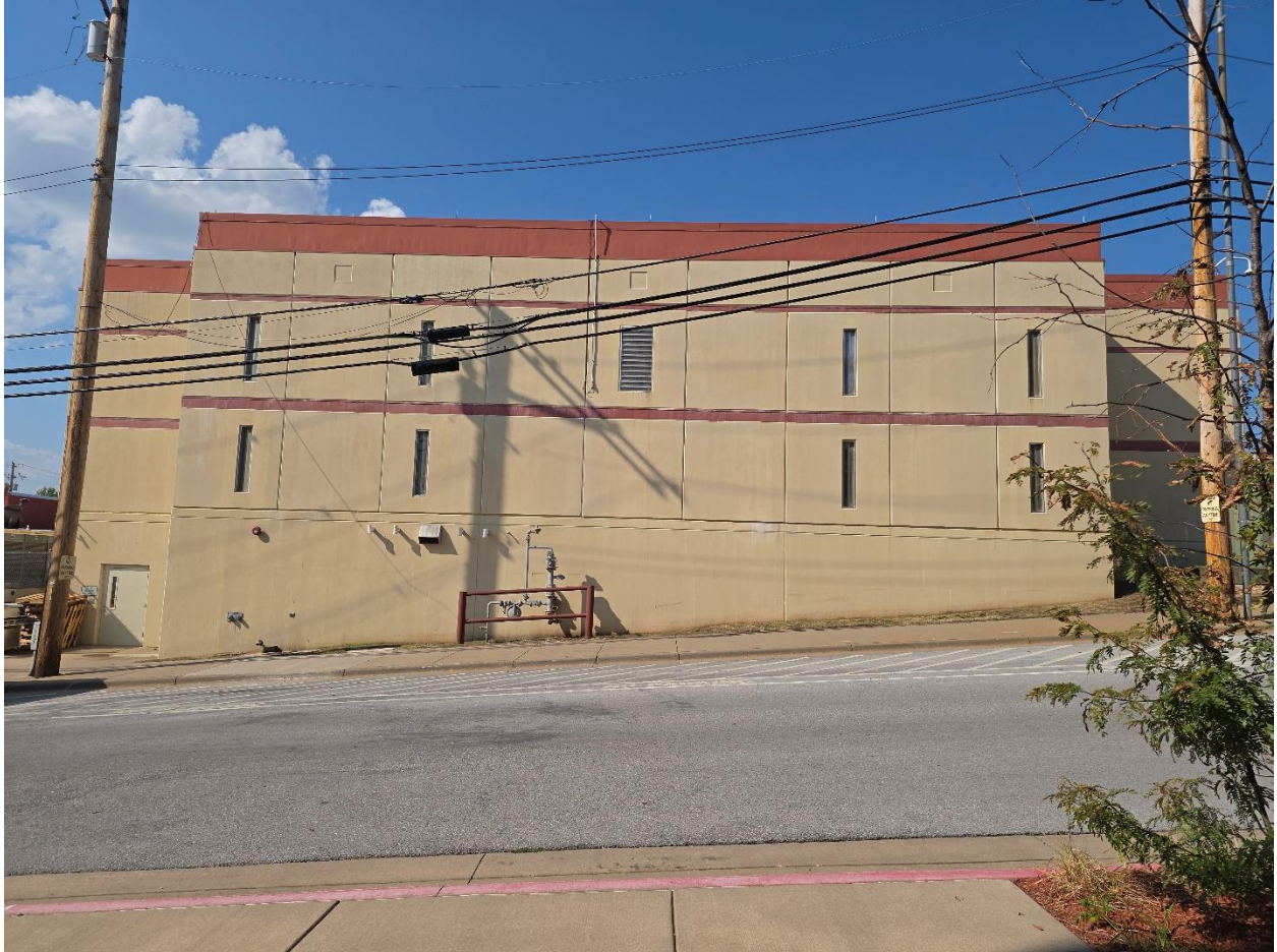
Back of Building
