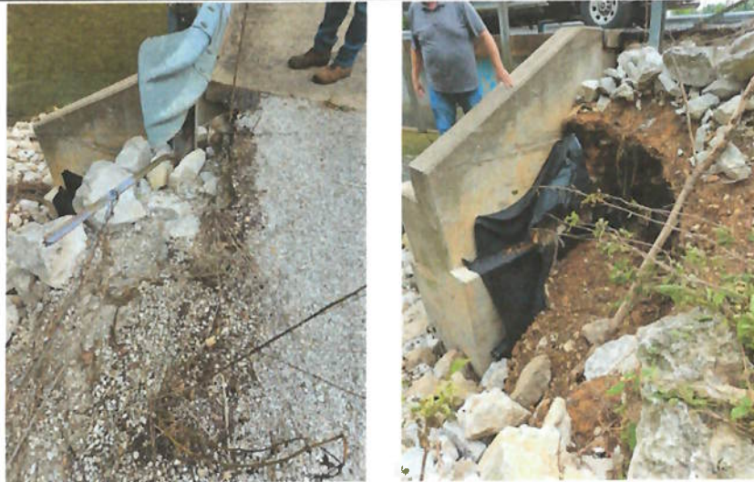
SHERROW BRIDGE (ARAPAHO RD), C1
