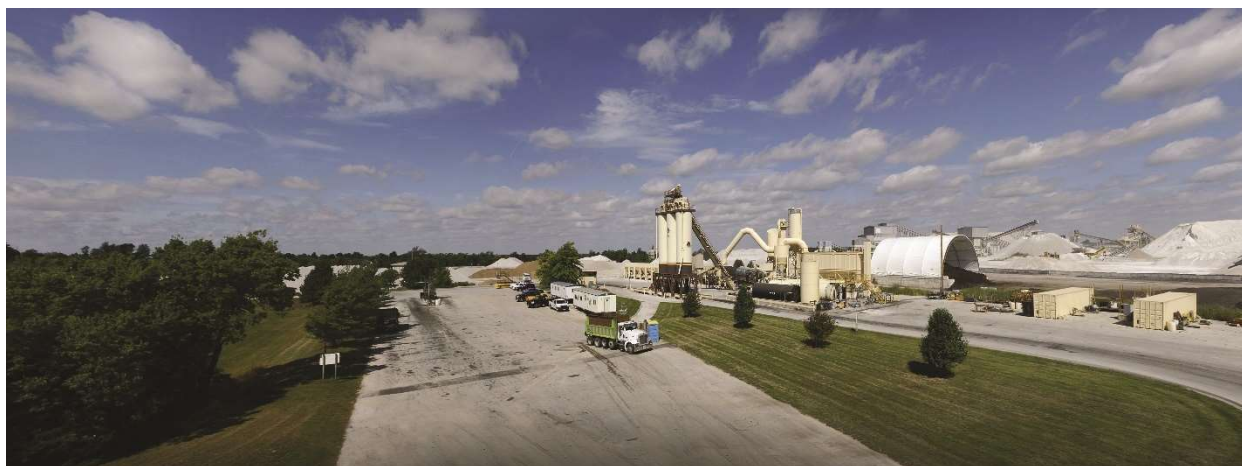
APAC-Central's asphalt plant in Willard, MO.
