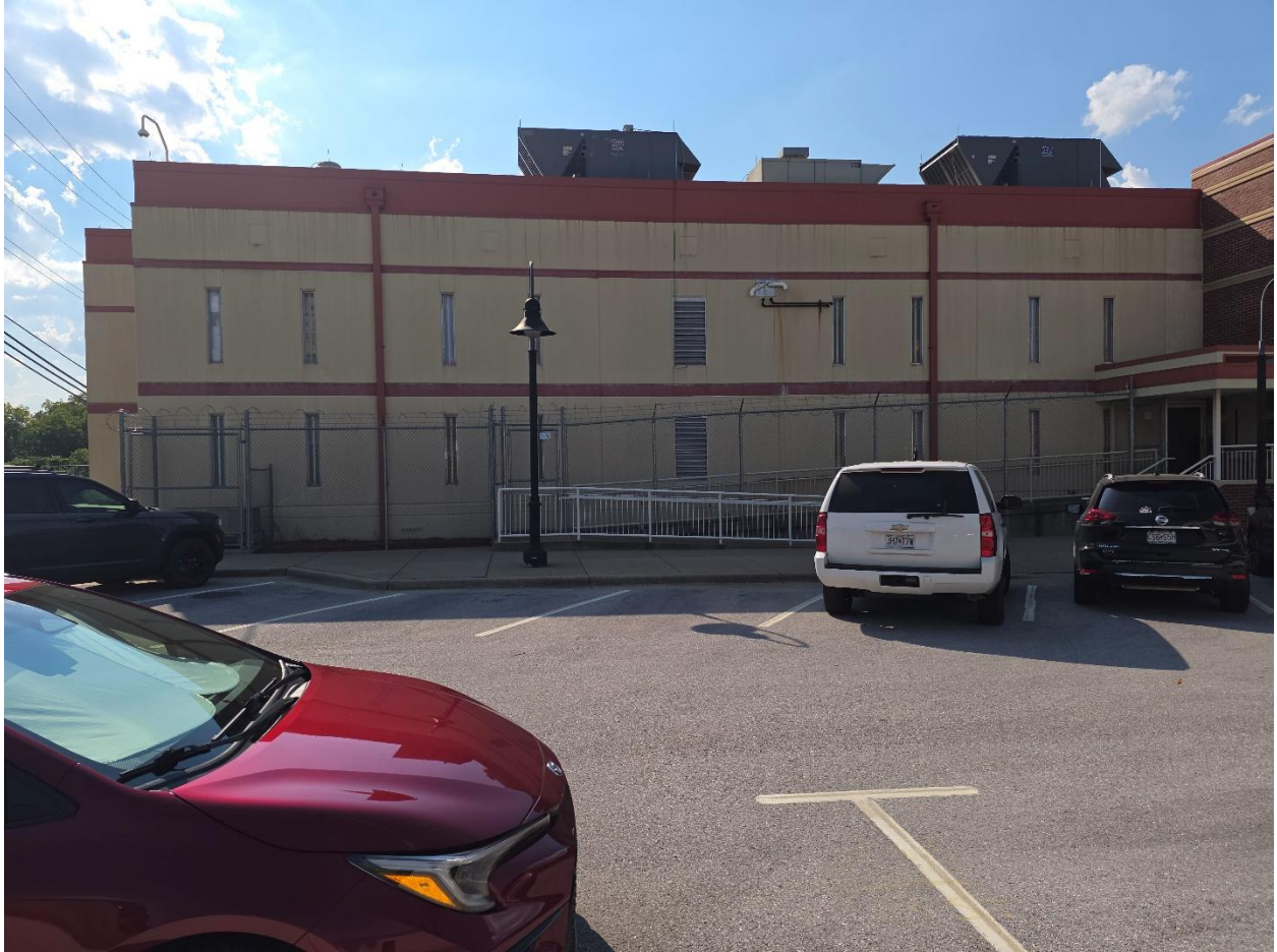
East side of the building
