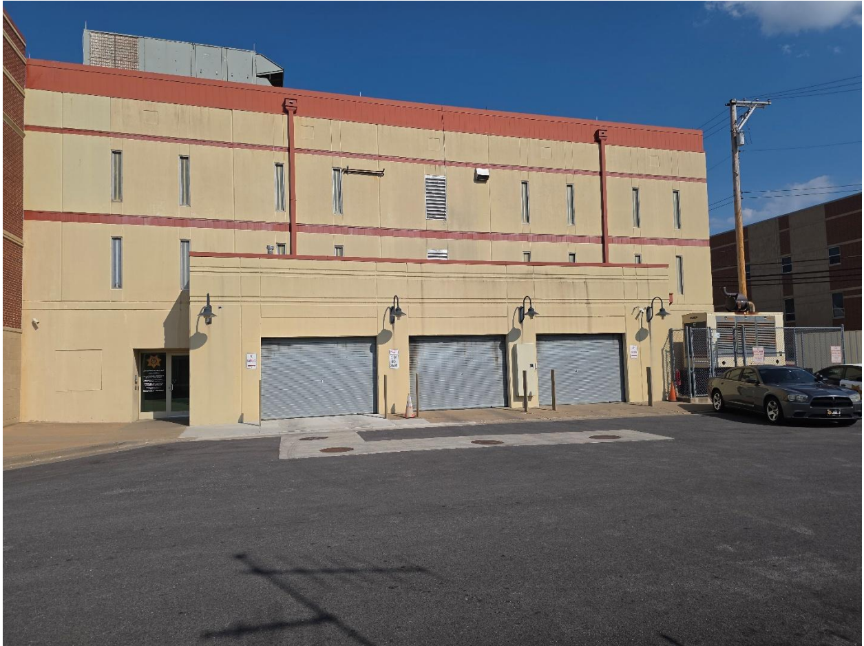
West Side of Building
