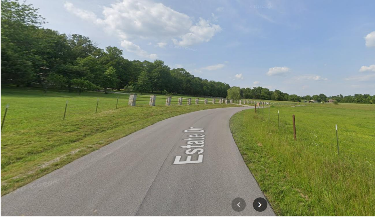
View of Estate Drive. 19 +/- feet in width
