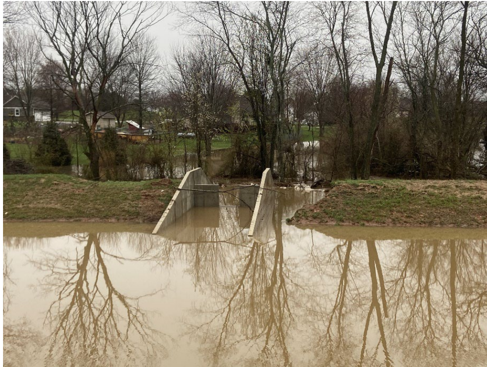
Figure 30. Excessive sedimentation in a losing stream that flows under Hemlock Road. The sediment is the result of inadequate erosion control measures from nearby residential development and road work. This losing stream contributes water to Fielden Cave, less than 1,400 feet away.
