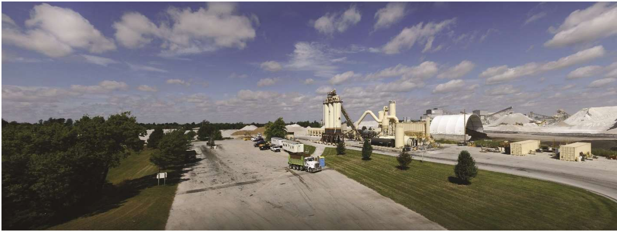
APAC-Central's asphalt plant in Willard, MO.
