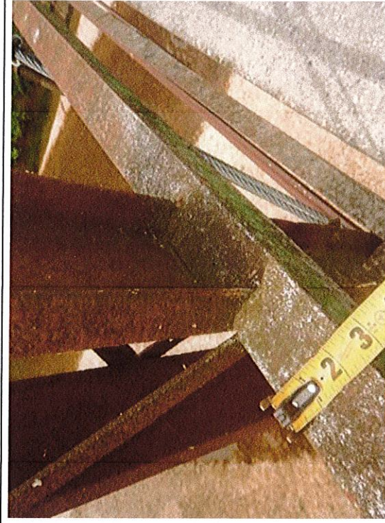
PHOTO 24 SPAN 4: Railing welded to vertical member (typical)
