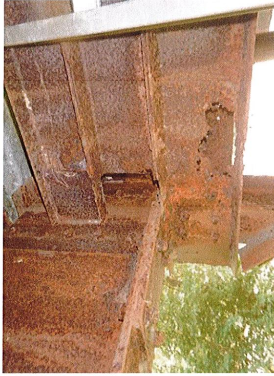
PHOTO 14 BENT 3 CAP, EAST END: 50% section loss to cap (typical north and south cap member)
