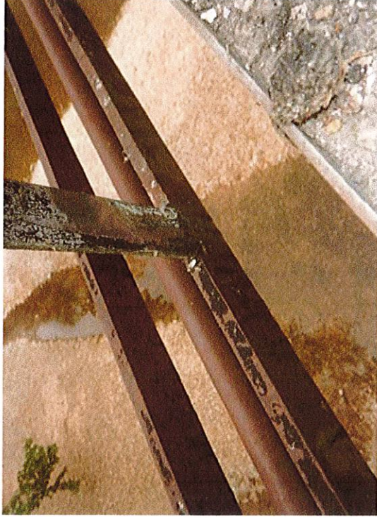
PHOTO 25 SPAN 4: Railing member welded to lower chord (typical)
