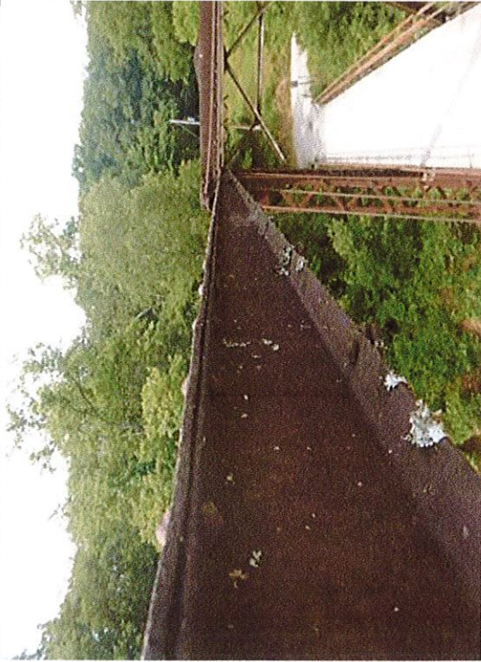
PHOTO 21 SPAN 4, UPPER CHORD: Typical minor pack rust jacking at upper chord panel points
