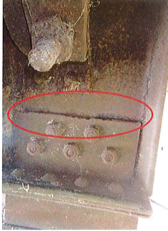
PHOTO 29 SPAN 4, WEST TRUSS, LO: Pin has 3/16" deep pitting on 1/4" of the pin circumference for 2/3 of pin length
