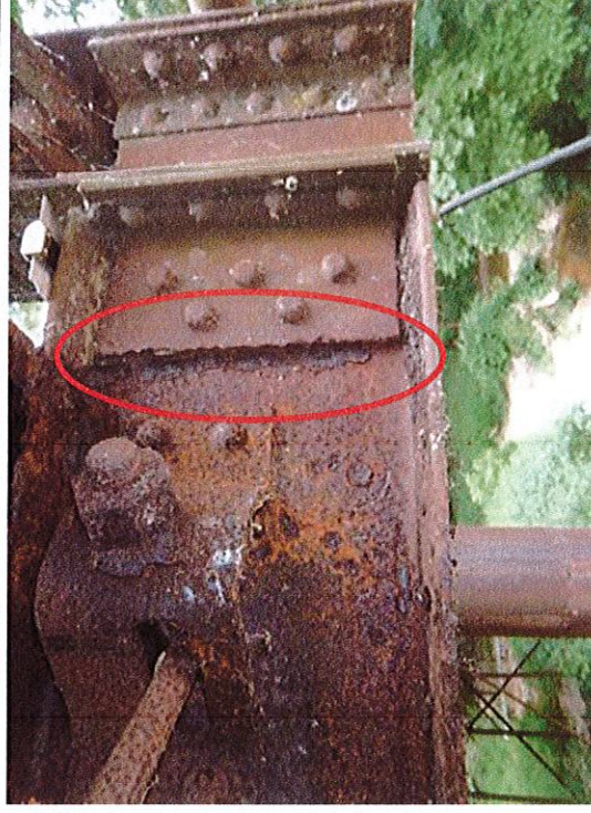
PHOTO 30 SPAN 4, FLOOR BEAM 1, EAST END, SOUTH FACE: Heavy section loss in web at end of clip angle connection
