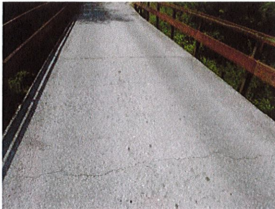
Typical asphalt deck surface
