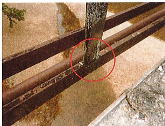
Thru Truss: Rail post welded to lower chord
