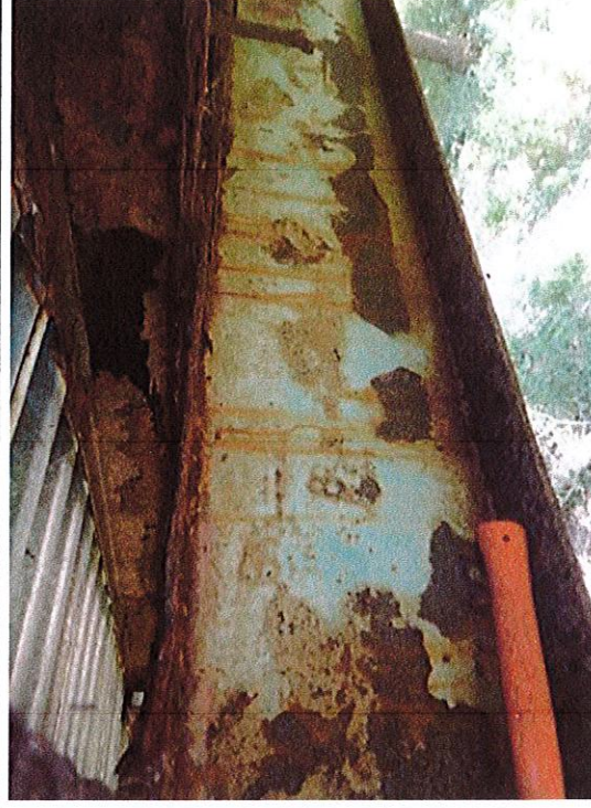
PHOTO 6 SPAN 1, WEST GIRDER, NEAR BENT 1: Heavy pitting with section loss for 7' length (9" height x 1/8" deep)
